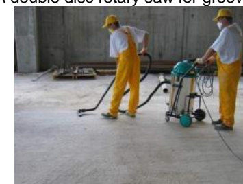
Industrial vacuum cleaner to remove dust on the surface
