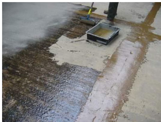
Priming with Sikafloor®-156 / -161
