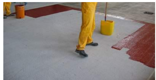
Priming with Sikafloor®-155 WN
