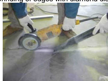
A single disc saw can do the job, but results are not as good
